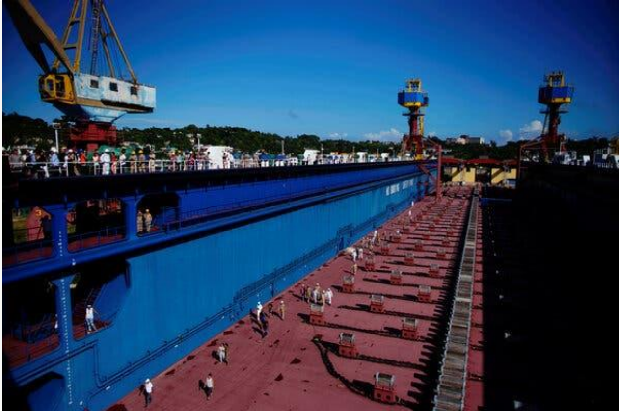
A floating dock in Havana for repairing Panamax-type ships, produced in China.
