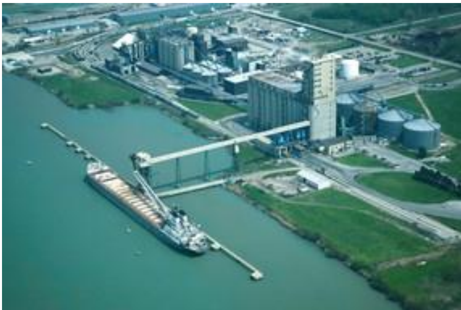
ADM Facility - at Port of Windsor
