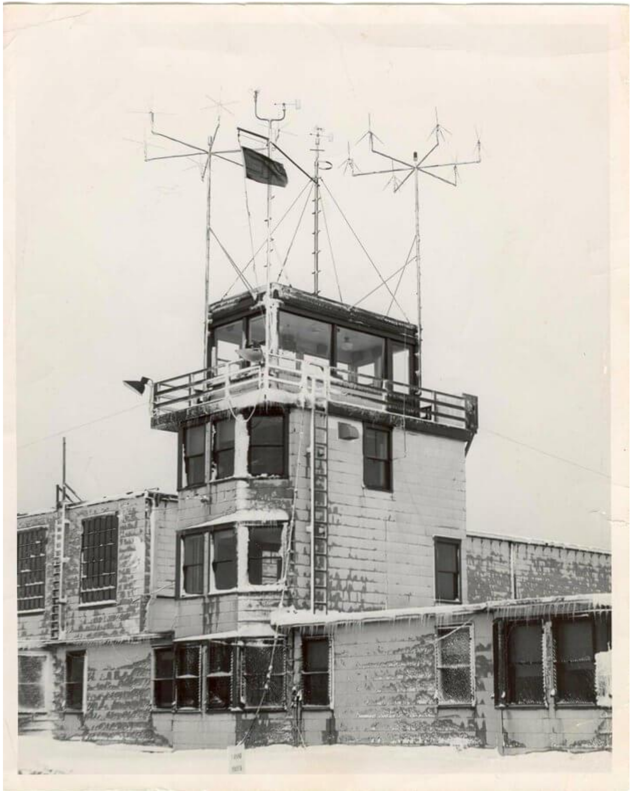
Canada's first air traffic control tower at Saint-Hubert Airport, circa 1940. Nav Canada/X Photo
